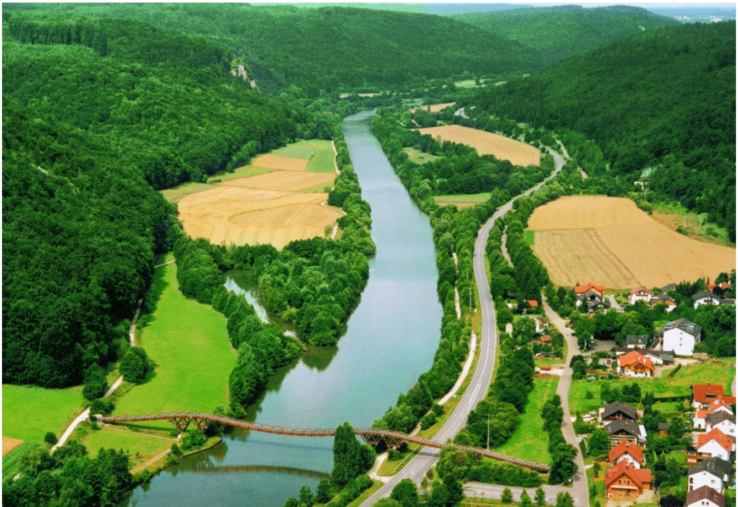
Rhine-Main-Danube Canal at Essing in Germany Construction □
