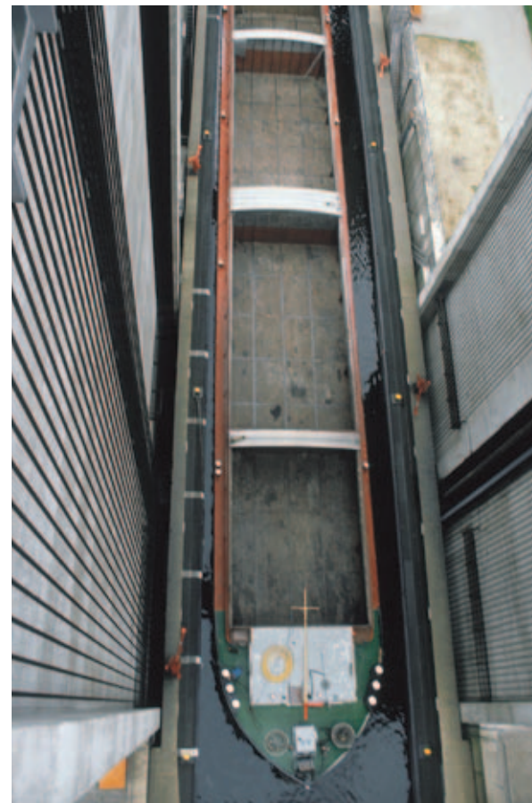
A double counterbalanced lift at Lüneburg on Elbe Lateral Canal, finished in 1975. Wire ropes, rope sheaves a counterweights are conveniently concentrated into four towers. The architecture of the lift proves that even design of a very high lift can steer away from the technocratic steel construction of the Niederfinow lift.
