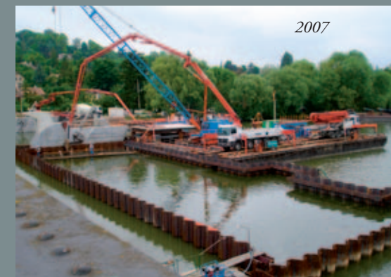
Construction of the new Oise dams with falling gates started at the dam Isle Adam, followed by the dam Pontoise.
