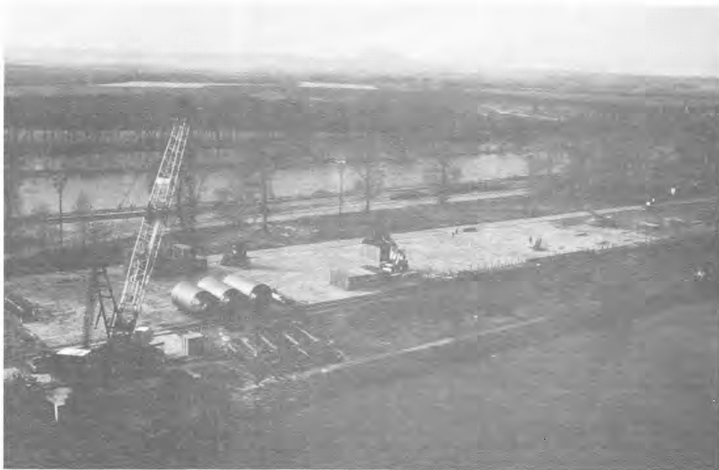
Fig. 1. Container terminal at Mělník – the first stage of construction. Overall view.
